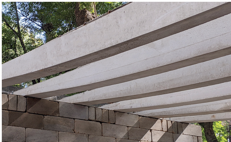
Prototype of a shape-optimized concrete floor system designed with Forma's generative software that saves 50% of concrete.
